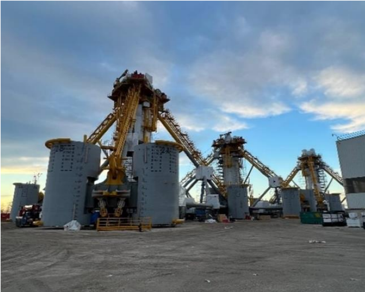
Image: Foundations under construction in Marseille for the Provence Grand Large
